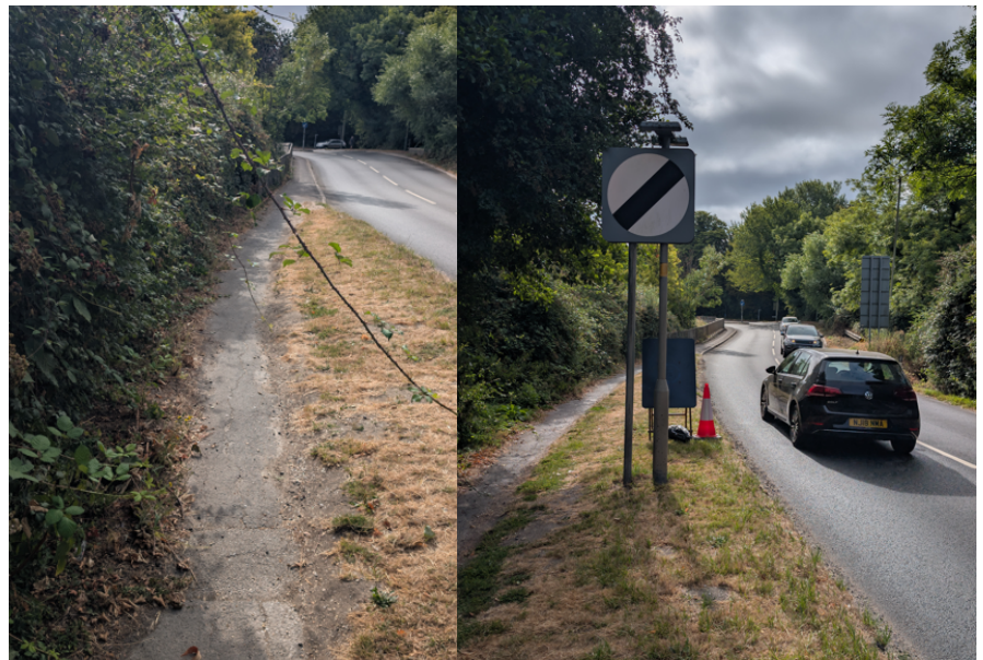
Pavement views from Hampton Park Roundabout towards St Thomas Bridge (L) just past the rail bridge, (R) approaching St Thomas Bridge.
